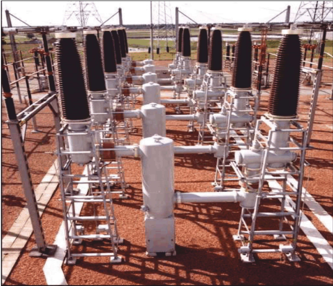
T155 Hybrid substation
